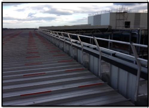
Quantum Parapet Rail Systems are a proven, low profile man-safe system which allows specifiers to provide lightweight yet durable roof access for maintenance purposes on any roof.
