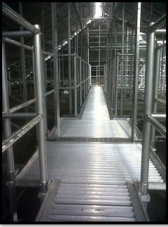
Quantum Internal Walkway is a proven, all aluminium fully welded roof access system which fixes to all Quantum access hatches. Manufactured in accordance with BSEN 516:2006, this product allows specifiers to provide lightweight yet durable roof access for maintenance purposes on any roofing system.
