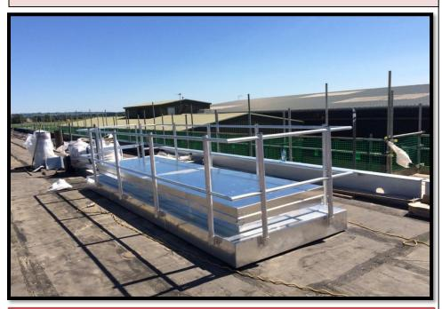
Quantum Hatchrail system is a proven, all aluminium fully welded roof access fall restraint system which fixes to all Quantum access hatches. Manufactured in accordance with BSEN 516:2006, this product allows specifiers to provide lightweight yet durable roof access for maintenance purposes on any roofing system.
