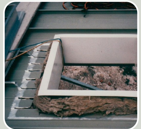
Paint removed from sheets prior to welding
