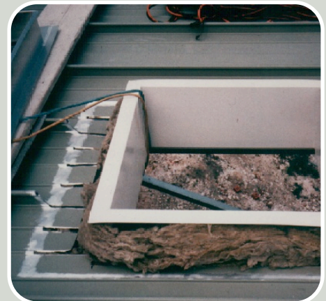
Paint removed from sheets prior to welding
